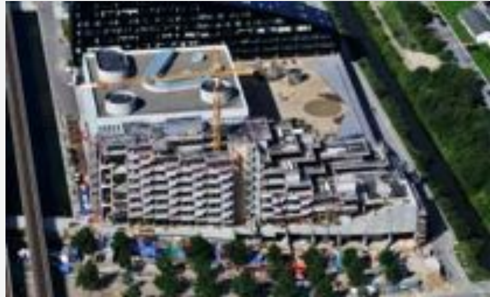
Ørestad School under construction.
