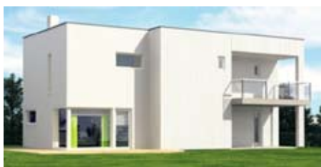
Demo house for energy efficiency Source: Norwegian Homebuilders Association (Boligprodusentenes Forening)
