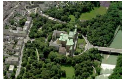
Projects from Siggi's career. From his time with Stirling Wilford: (top) Neue Staatsgalerie, Stuttgart; From Léon Wohlhage Wernik: (middle) Caleido offices in Stuttgart – visualisation; (above) Bavarian state parliament with extension cube lower centre – photo montage; (below) Health Campus North Rhine-Westphalia, Bochum – visualisation Sources: Neue Staatsgalerie, Muskiproz, 2004 (GNUFDL); all others Léon Wohlhage Wernik
